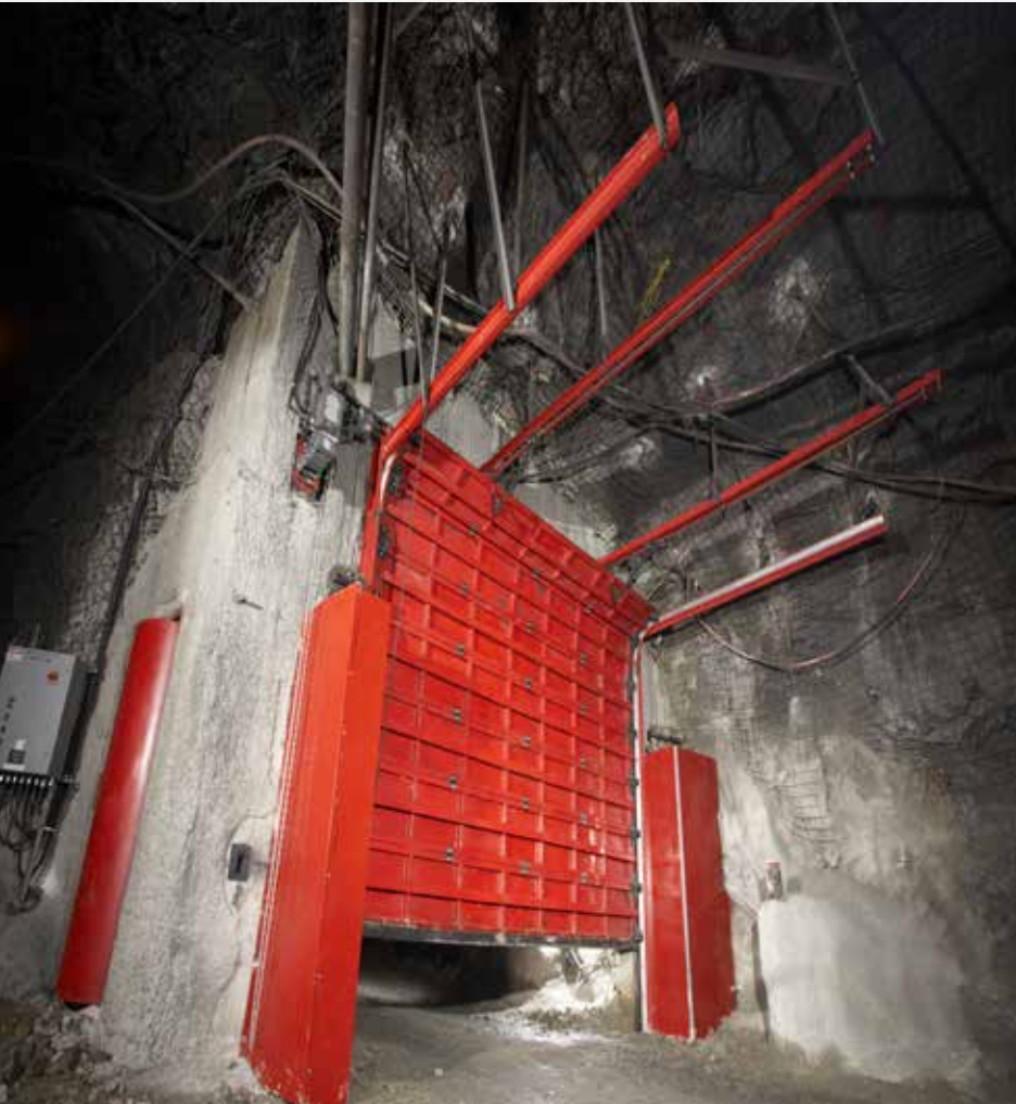
An installed high pressure steel sectional mining ventilation door system, identical to the doors that Innu-Inuit PDI has supplied to the Vale underground project. (PDI photo)
