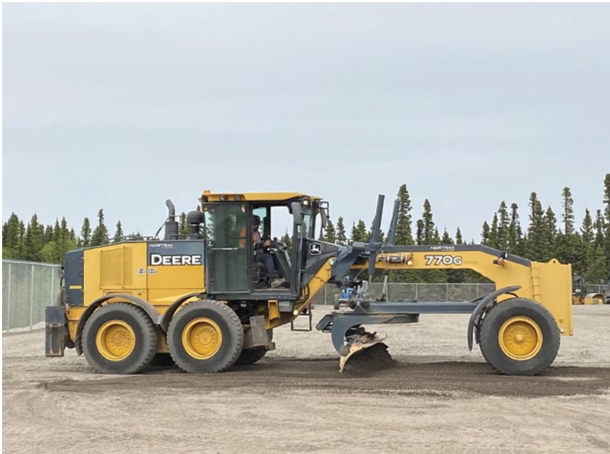
The acquisition substantially adds to NCI's ability to engage in heavy civil work. (Photos: DJ Elliott)
