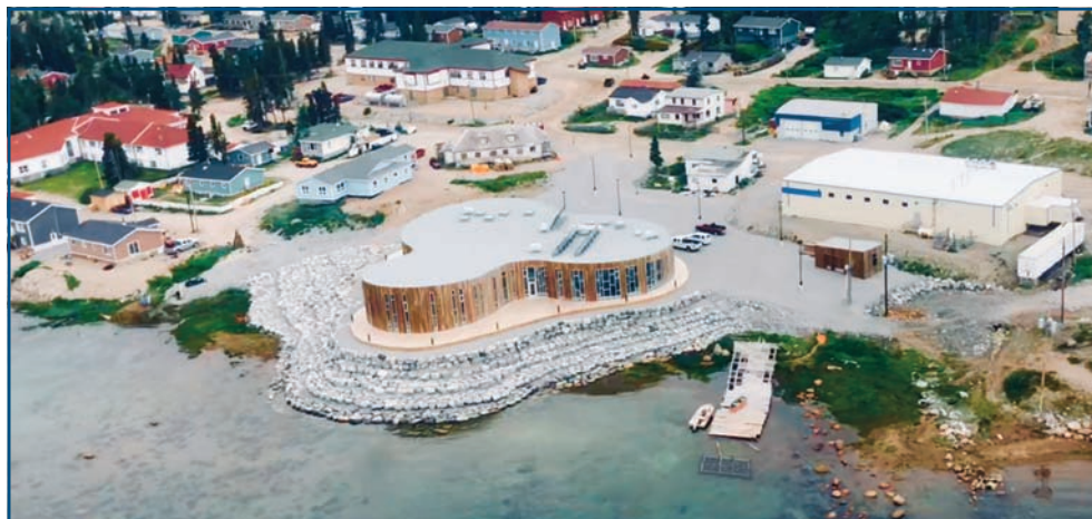
The Illusuk Centre in Nain is expected to open in late 2018. The Centre will house permanent exhibits, an audio-visual/performing arts theatre, café, gift shop, and several offices. It will also be a place where Inuit culture, language, traditions, stories and experiences will be shared and celebrated.
