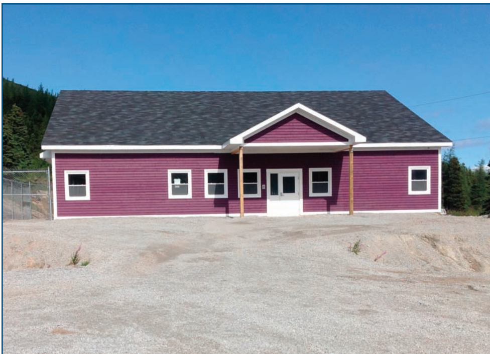
The Nain Transition House was built by an all-Nain labour team, evidence of the skill set being developed at NCI. The project superintendent was Russ Petten.
