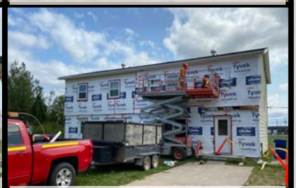
Exterior Renovation Happy Valley-Goose Bay
