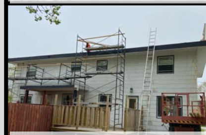
Roofing Job Happy Valley-Goose Bay
