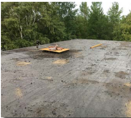
Modular bitumen roofing involves cold application of three layers of waterproof protection. The photos show the progression from exposed roof through to the finished stage. (Tom Lyall photos)
