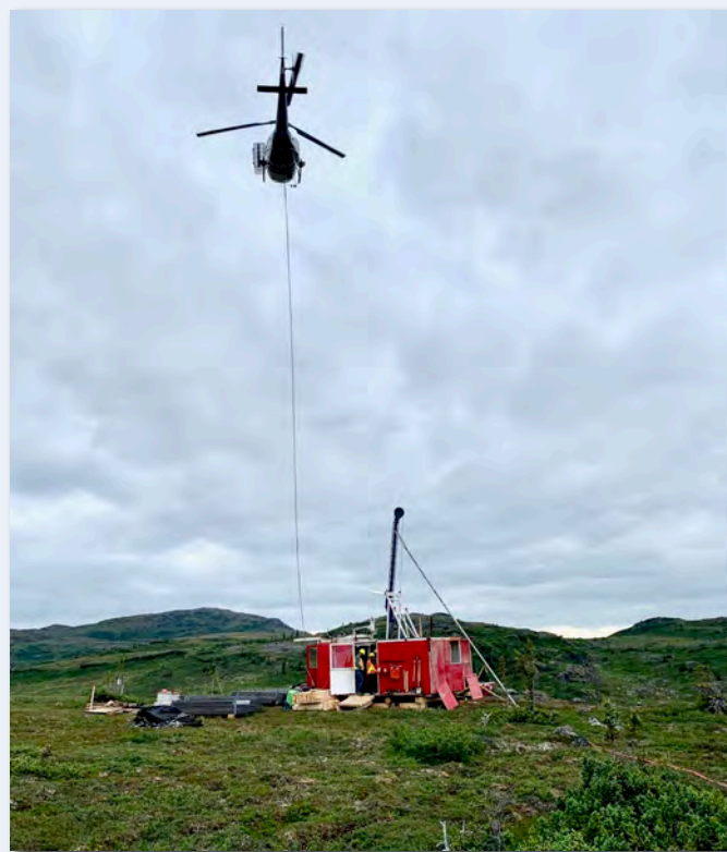
The pilot places drilling equipment and drill pipe in place with a longline.
