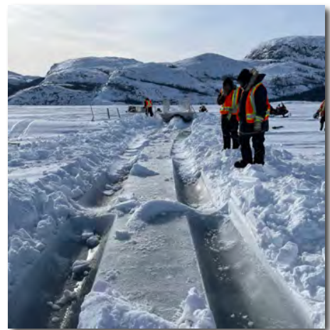
The Sikuliatsiuk crew arrives on Anaktalak Bay to begin the work of placing pontoons across the ship's track. The pontoons are heavy. Wenches and snowmobiles are required to position them across the open water to provide safe crossing for snowmobilers. The Umiak I has made three trips this winter, on January 22, February 28, and March 23. The next scheduled trip after March is May 22.
