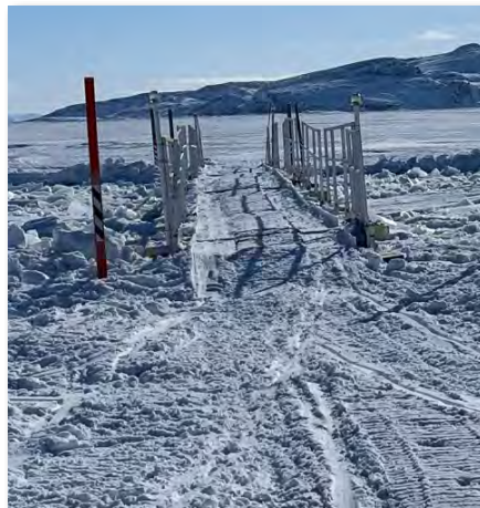
Cables are attached to the pontoons as the work begins to drag the buoyant steel structures across the opening created by the Umiak I. Slowly, the pontoons are pulled across the open water. Markers are placed to alert snowmobilers to the safe crossing areas and guardrails installed to ensure safety while crossing. The pontoons have to be removed for the ship's outbound journey and then reinstalled until the next trip.
