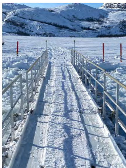
At left, the Sikuliatsiuk crew uses winches and snowmobiles to position the steel pontoons into place across the ship's track. At right, the pontoons are in place, creating safe passage for snowmobiles. (Stephanie Angnatok photos)
