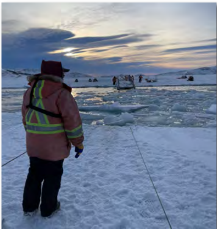
Cables are attached to the pontoons as the work begins to drag the buoyant steel structures across the opening created by the Umiak I. Slowly, the pontoons are pulled across the open water. Markers are placed to alert snowmobilers to the safe crossing areas and guardrails installed to ensure safety while crossing. The pontoons have to be removed for the ship's outbound journey and then reinstalled until the next trip.
