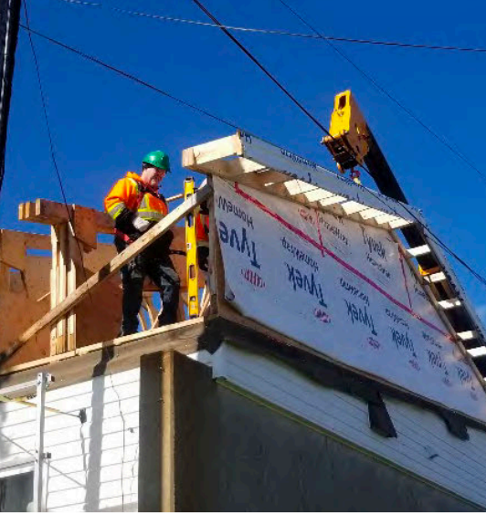
(Left to right) An NCI crew at work replacing the roof on a NL Hydro seven-unit residential building in Churchill Falls. Centre, a residential roofing job in Rigolet, part of the Nunatsiavut Government's Home Repair Program. Right, roof replacement on the NL Hydro plant at St. Anthony. (NCI photos)
