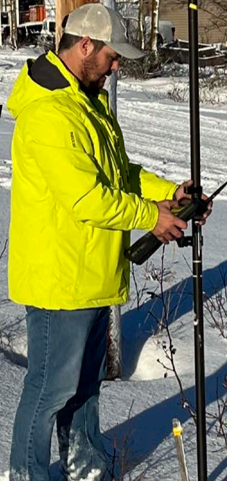
Ryan Snow, NCI's Senior Project Manager, surveying the site of the Nunatsiavut Government's new Community Education Centre in Makkovik, on December 12. NCI was the successful bidder for Phase One of the project, which includes the sub-grade. Tenders for Phase Two, the actual building, are expected to be released in the spring. (Ryan Snow photos)
