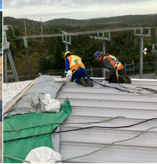
(Left to right) An NCI crew at work replacing the roof on a NL Hydro seven-unit residential building in Churchill Falls. Centre, a residential roofing job in Rigolet, part of the Nunatsiavut Government's Home Repair Program. Right, roof replacement on the NL Hydro plant at St. Anthony. (NCI photos)
