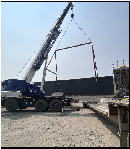
Left, crane operators, riggers, and truck drivers were involved in lifting a conveyor gallery for the Reid Brook conveyor system. Centre, a TSI crew assists in unloading equipment for the expansion project from an aircraft. Right, heavy equipment operators sort ore prior to the ore being sent to the crusher.
