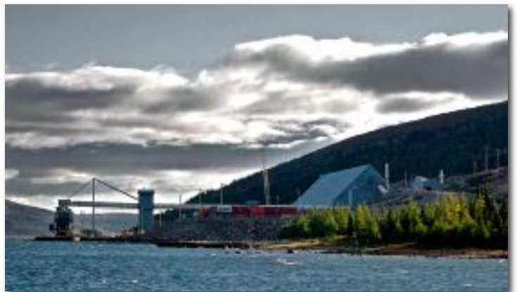
TSI provides sites services at Voisey's Bay, including loading and unloading at the dock.
